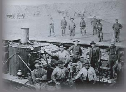
The First Open Pit
